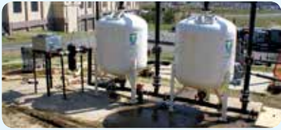
Dual D54 dryers (left) are used at a landfill to remove moisture from low pressure methane. A D36 dryer (right) is used to remove moisture from compressed air on a steel grit recycling trailer.
